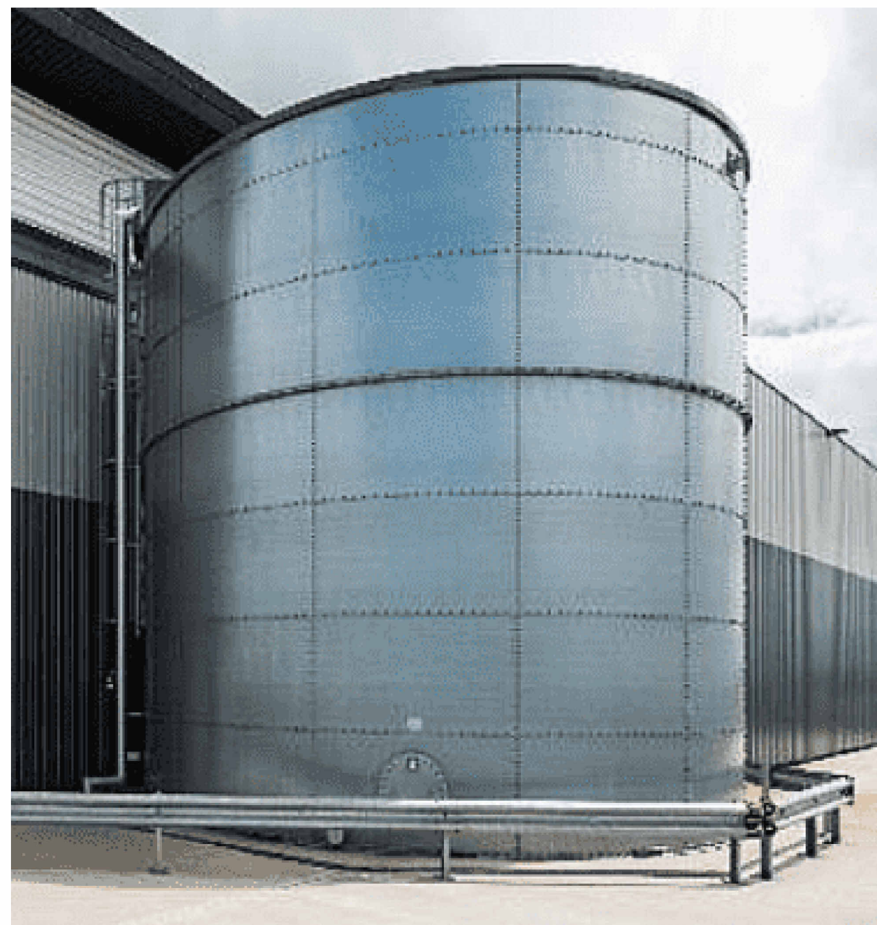
TYPICAL PROCESS & FIRE WATER STORAGE TANKS (N.T.S.)
